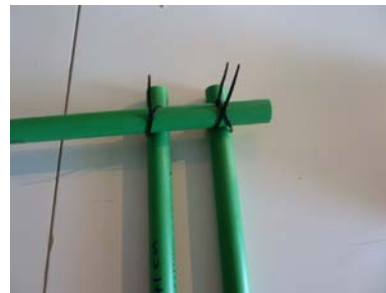
Figure 2. In this picture we can see how we can keep on fastening pipes together in order to construct the frame of the platform.
